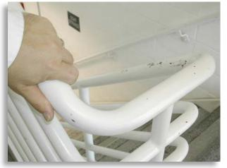
This handrail provides continuous gripping contact from the top floor to the bottom landing.
