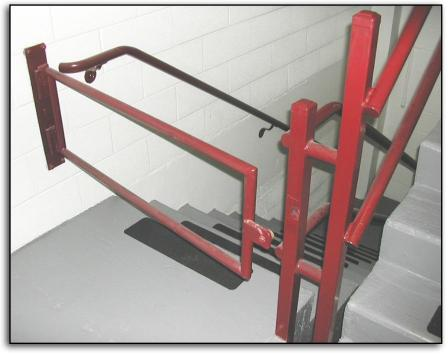
This barrier is intended to prevent a person from inadvertently walking below the level of exit discharge.
