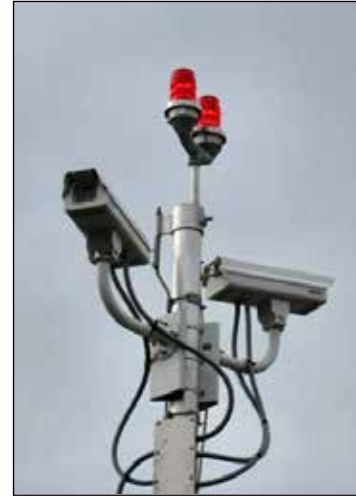
Figure 6-34. Weather Camera (WCAM) Pole
