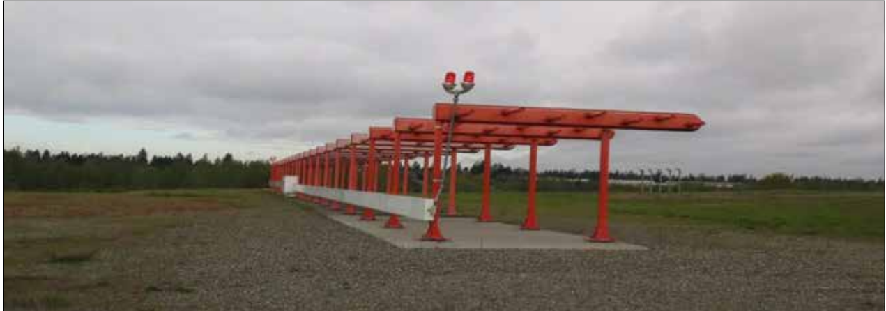
Figure 6-22. LOC 14-Antenna Array
