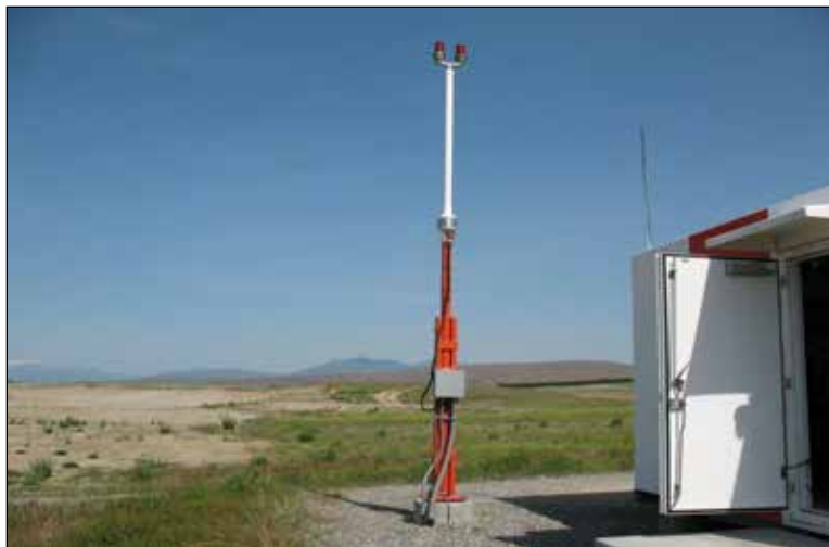
Figure 6-25. DME Antenna
