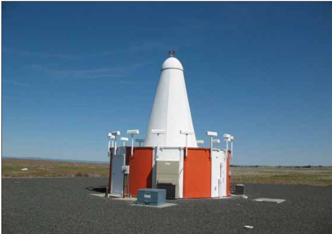
Figure 6-28. Terminal VOR (TVOR) Facility
