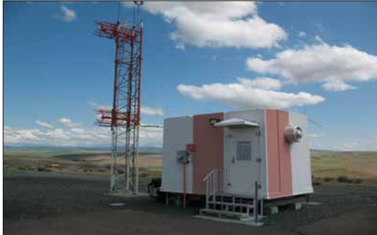
Figure 6-24. GS Antenna and Equipment Shelter
