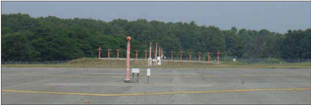
Figure 6-15. Approach LDIN Facility
