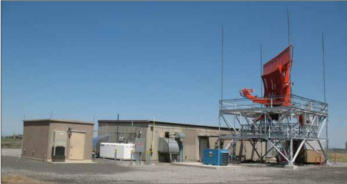
Figure 6-5. ASR Steel Tower (17 feet (5 m) high)
