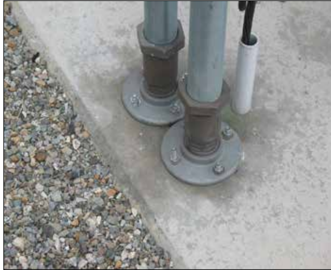
Figure 6-2. Two Frangible Connections
