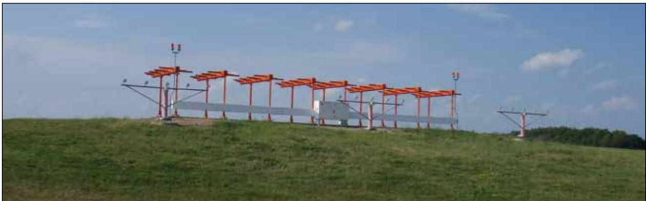
Figure 6-21. LOC 8-Antenna Array
