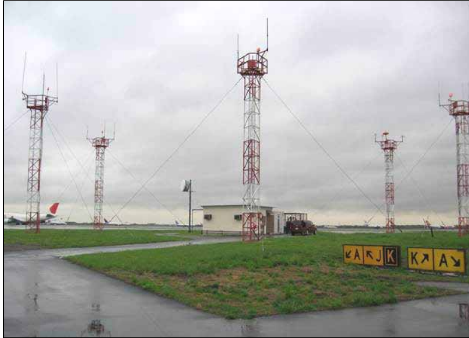
Figure 6-4. RTR Communication Facility
