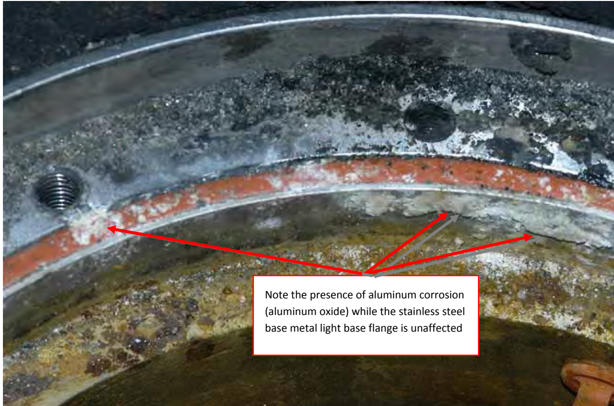
Figure 11. Stainless Steel Light Base with Aluminum Light Fixture Removed
