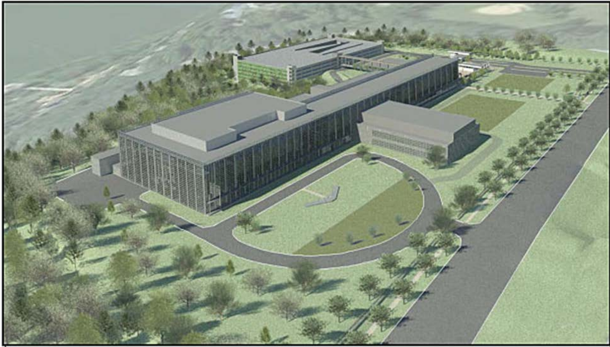
Figure 4: Illustrated view of the proposed concept for the Intelligence Community Campus-Bethesda, looking northwest (the installation continues to front Sangamore Road, which runs diagonally across the right side of the illustration). Note that the illustration does not reflect the current proposed size and location of the parking garage or alignment of the access road.
