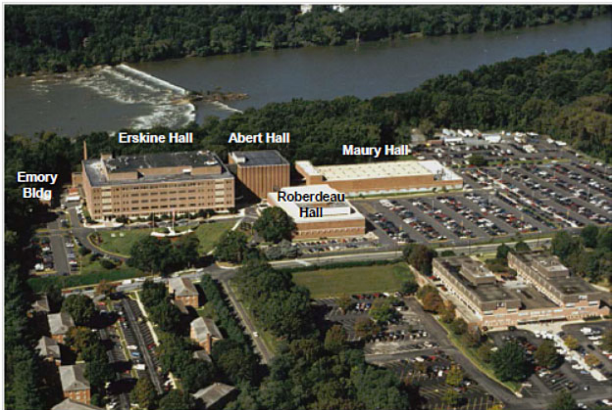
Figure 3: Birdseye view of the existing condition of the installation, looking west (the installation fronts Sangamore Road, which runs through the center of the photograph).
