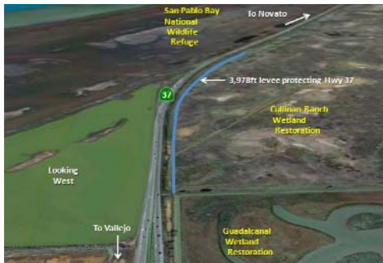
San Pablo Bay Levee Rehab to Restore Tidal Flow
