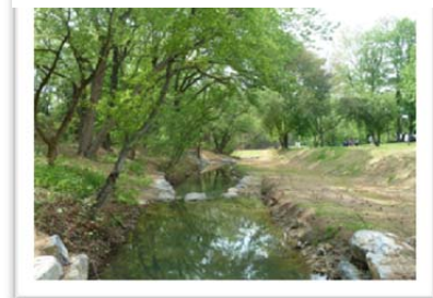
Watts Branch – After restoration
