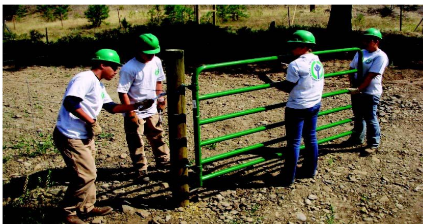
Turnbull NWR Youth Conservation Corps crew installing a new gate.
