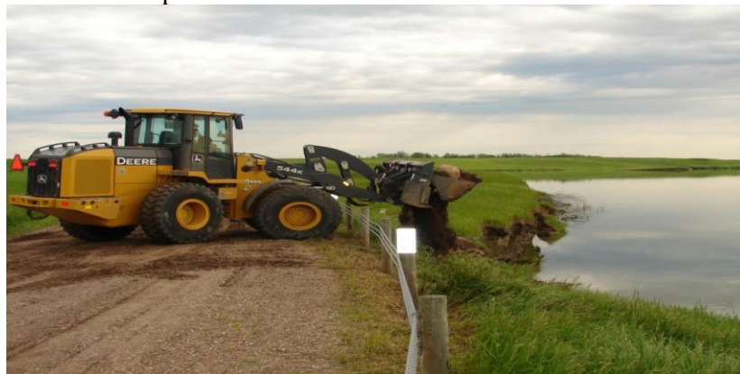
Heavy equipment used in dike repair at Audubon NWR
