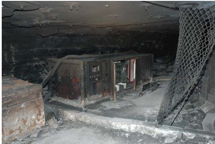
Figure 8. Former location of stopping at the electrical installation.
