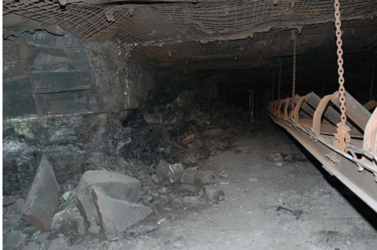
Figure 6. Location where belt structure was installed after removal of a stopping.
