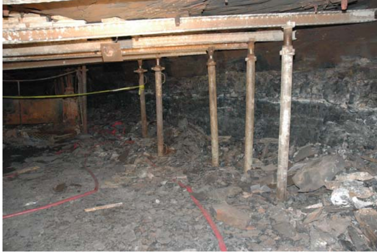
Figure 4. Area inby No. 7 Belt tail pulley. (Roof support was installed post-accident.)
