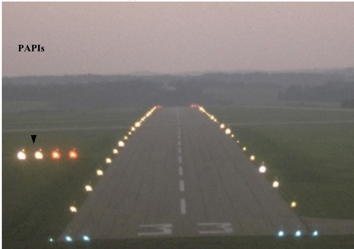
Figure 3. PAPI Light Fixture showing glide path information
