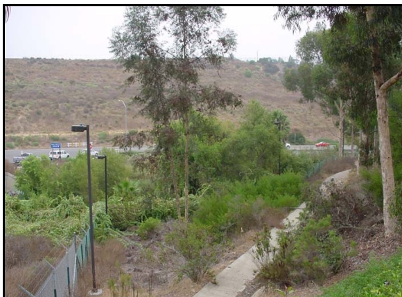
Photograph 2-4. Culvert Used to Collect Runoff and Reduce Erosion along the Eastern Slope
