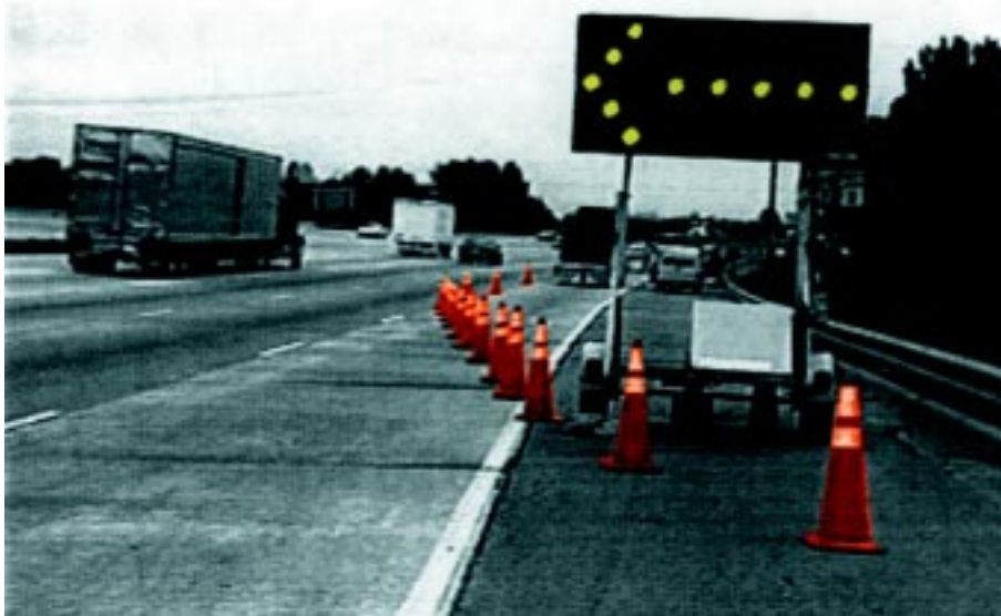
Proper taper setup for closing first lane and shoulder.
