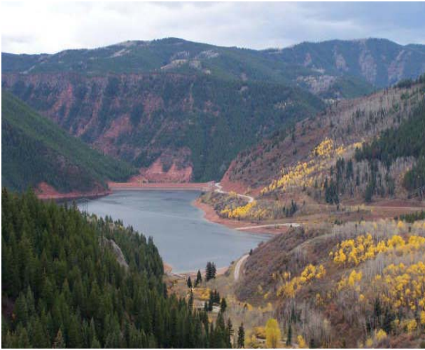
Ruedi Reservoir provides water to the west slope to make up for water diverted to the east slope.
