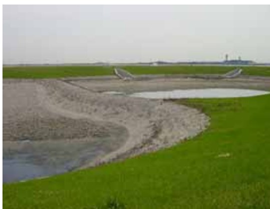
This storm water basin was designed to drain within 48 hours following a major storm event (the design storm). The rip-rap lining helps prevent vegetation growth and bird use of the pond (photo courtesy FAA).
