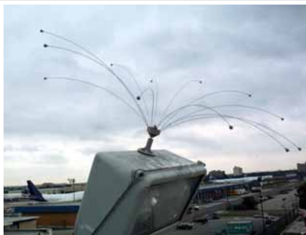
Light posts and other structures in taxicab lots at airports can be fitted with anti-perching devices to discourage gulls and other birds from using the area. Feeding of birds should also be prohibited on airport property.
