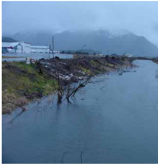
Bodies of open water adjacent to airports, such as this drainage canal, are often magnets for waterfowl and wading birds. Note the shallow slope that allows birds easy access in and out of the water. Such canals should be covered if possible or diverted away from the airport (photo by E. Cleary, FAA).
