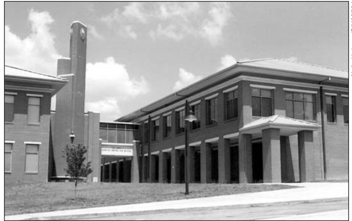
Daylighting and exterior shading are featured in the design of the U.S. Army Chaplain Center and School at Fort Jackson, South Carolina, to reduce electrical and cooling loads.
