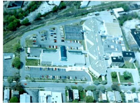
Exhibit 4b: Aerial View of Dutchess County Jail Facility, Poughkeepsie, NY
