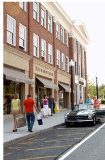
Exhibit 9: Mashpee Commons, in Cape Cod, created pedestrian places within its retail center.
