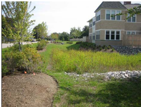
The town of Wells has experience with infiltration approaches. The new medical center on Rt. 109 has a good example of a swale that manages stormwater on-site.
