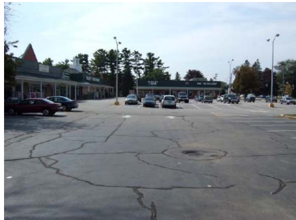
Exhibit 25: Wells Corner shopping area parking lot
