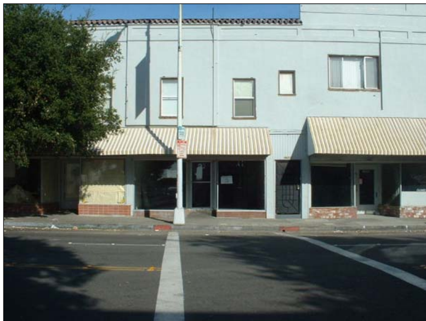
Figure 6.1A View of existing street. Source: Kimley-Horn and Associates Inc.
