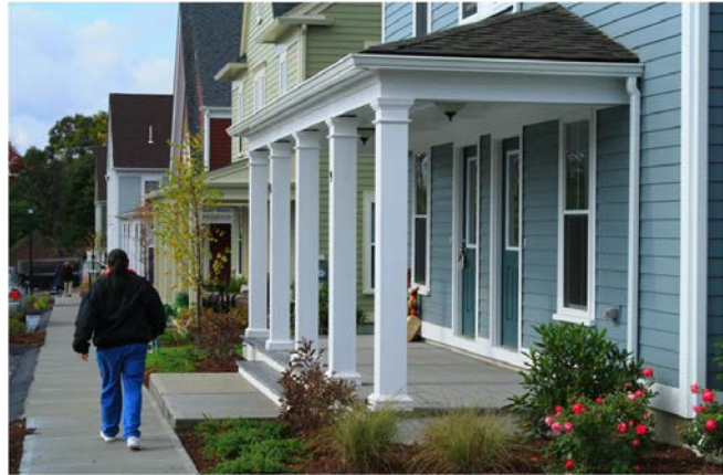
The Sweetbriar Development includes 47 new affordable homes for rent in Barrington, RI. Photo courtesy of Union Studio Architecture & Community Design.
