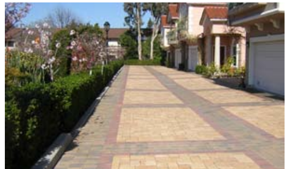
Figure 4-12: This residential driveway uses pervious pavers in San Mateo County, California.
