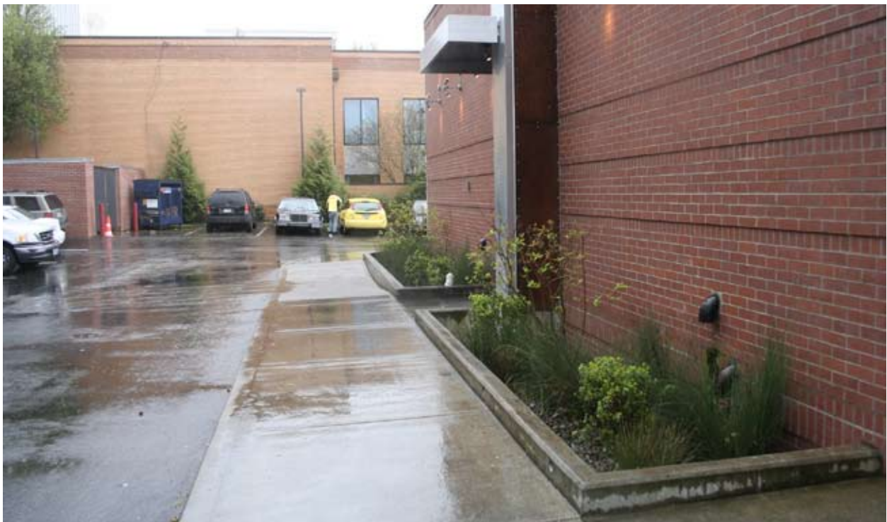
Figure 4-38: A stormwater planter accepts stormwater runoff from a fast food restaurant’s rooftop.
