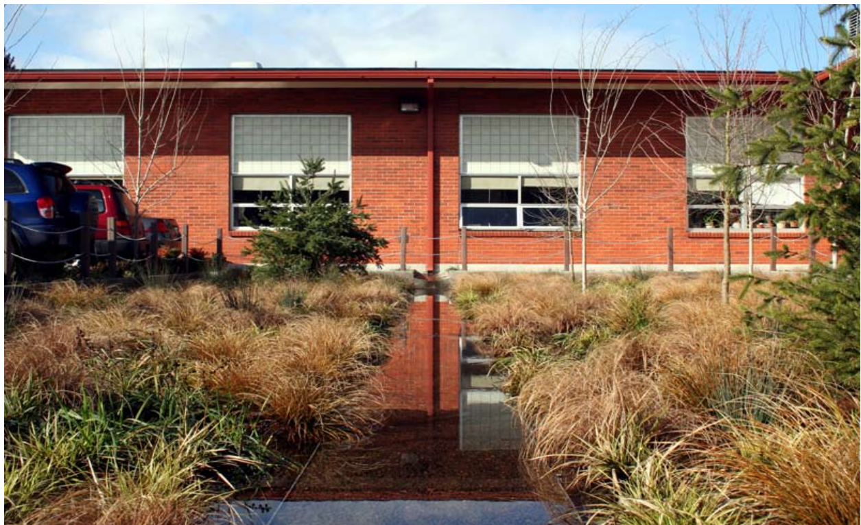
Figure 4-45: A large infiltration garden accepts stormwater runoff from a middle school's rooftop.
