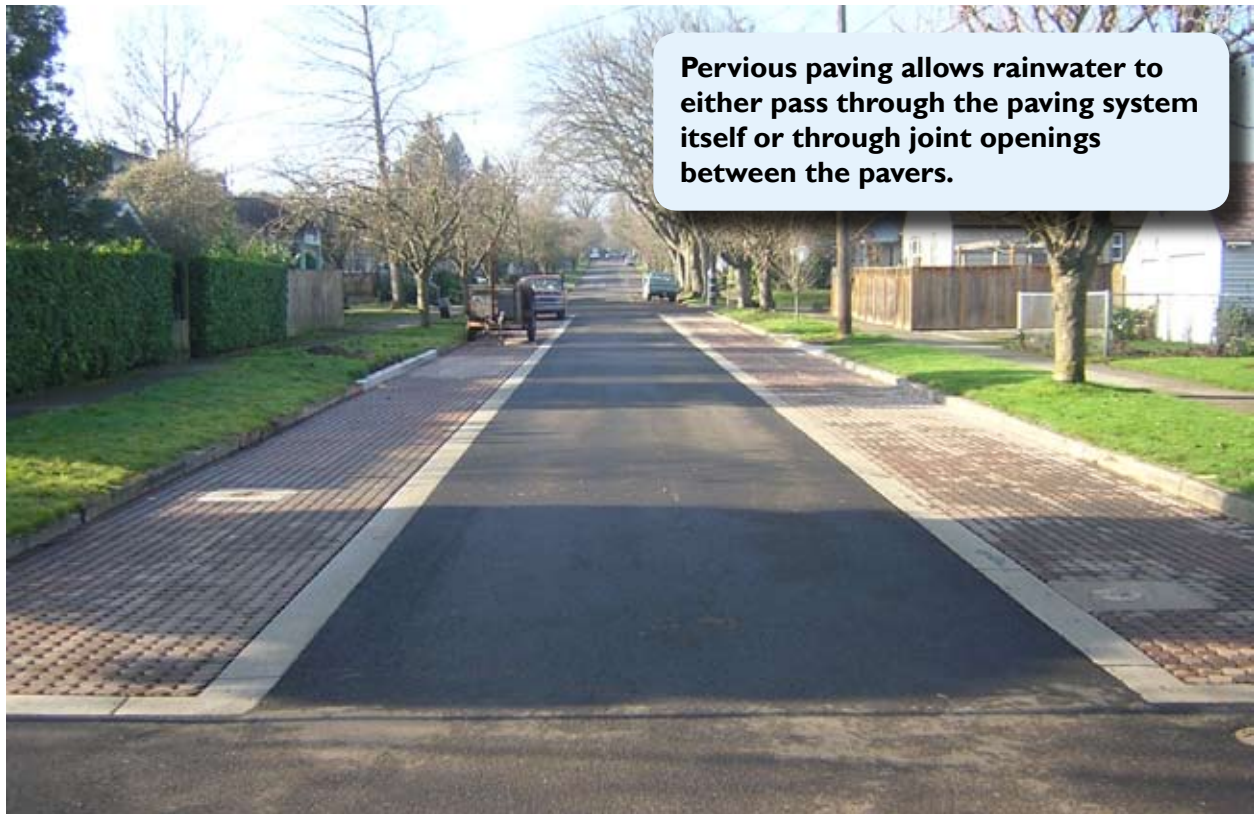
Figure 4-6: Pervious paving used in the parking zone on a residential street in Portland, Oregon.
