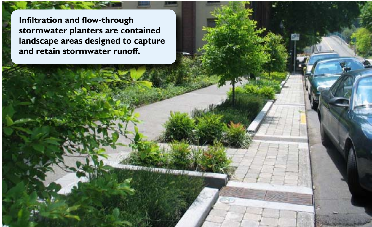
Figure 4-32: Stormwater planters are used to infiltrate stormwater runoff on a downtown street in Portland, Oregon.
