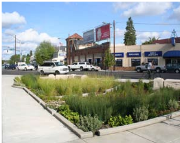
Figure 4-42: A triangle-shaped infiltration garden retrofitted along a busy arterial street.
