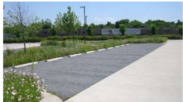
Figure 4-13: A plastic grid system filled with gravel provides the structural strength to support a vehicle.
