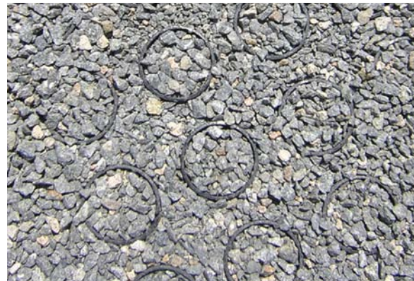
Figure 4-19: A close-up view of gravel paving within a reinforced plastic grid system.
