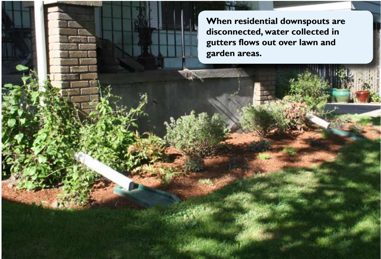
Figure 4-57: Roof downspouts can be easily disconnected and allow runoff to flow into surrounding landscaped areas.
