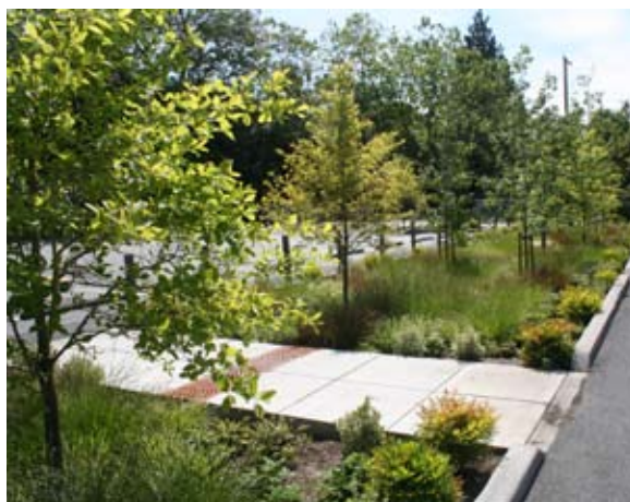
Figure 4-43: An infiltration garden retrofitted within a middle school's parking lot.
