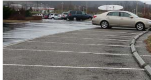
Figure 4-11: The difference between drainage on pervious asphalt and impervious asphalt is evident in this photo.
