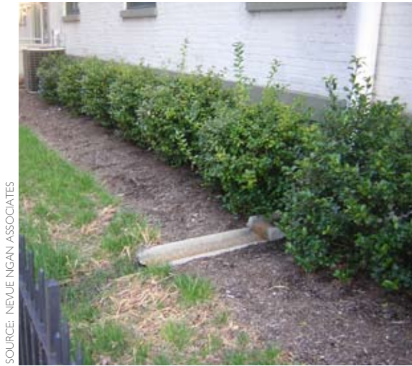
Figure 4-58: An office building in Covington has disconnected roof downspouts that allow water to flow into a landscaped area.
