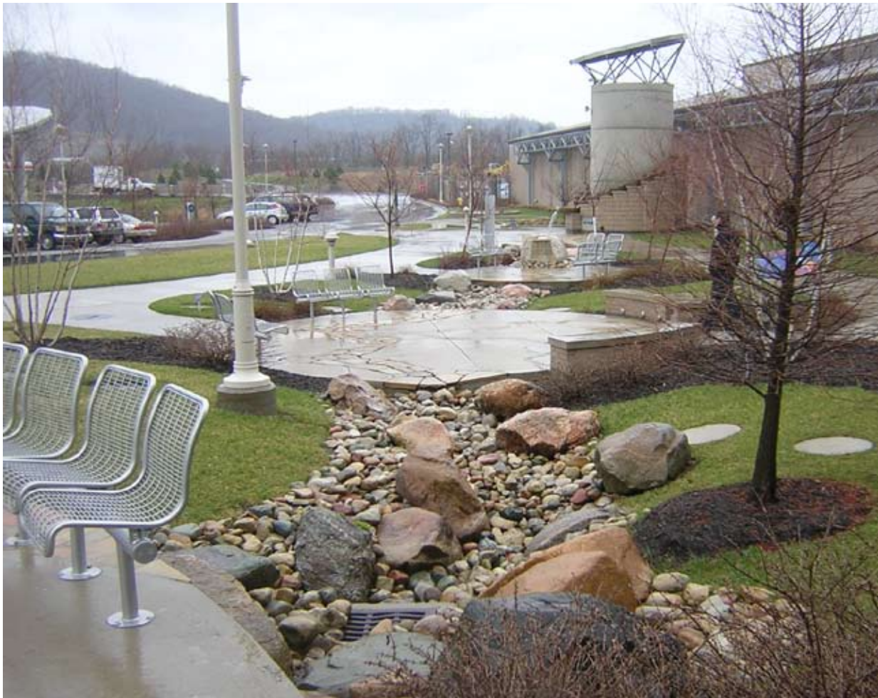
Figure 4-31: This stormwater swale at the Sanitation District No. 1 of Northern Kentucky headquarters collects runoff from the building's rooftop.
