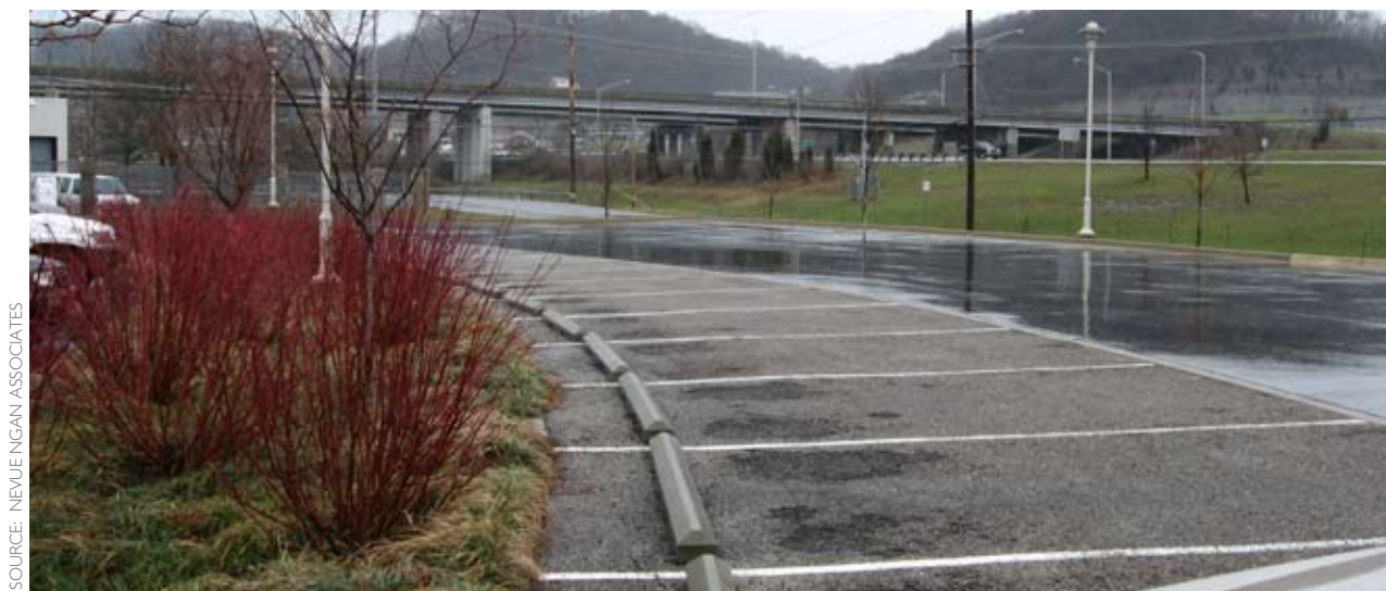
Figure 4-17: Pervious asphalt in the parking stalls at the Sanitation District No. 1 headquarters.
