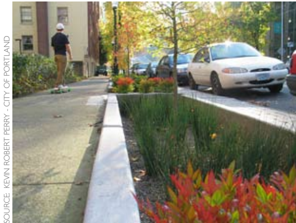
Figure 4-34: An urban street infiltration planter.
