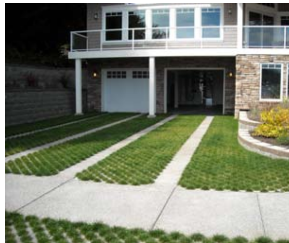
Figure 4-20: Grass paving installed in a residential driveway.
