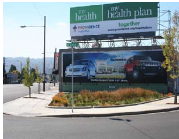
Figure 4-56: A large stormwater curb extension retrofit along a busy arterial street.
