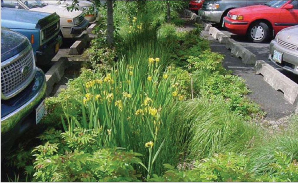
Figure 11: Parking lots can use low-impact drainage infrastructure to collect stormwater and protect water quality. Using native plants can make the parking area more attractive. (Source: ICF)
