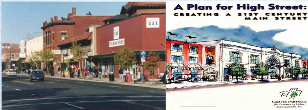
Exhibit 2.3: Campus South Gateway project, Columbus, Ohio. Photos from Campus Partners website.
