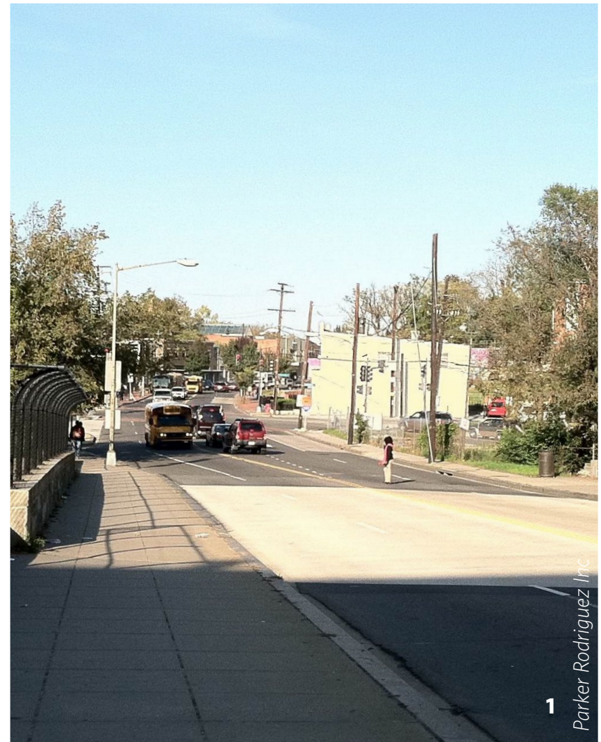
Figure 21: MLK Avenue has four lanes with sidewalks on both sides of the street between eight and 10 feet wide at the station area.
