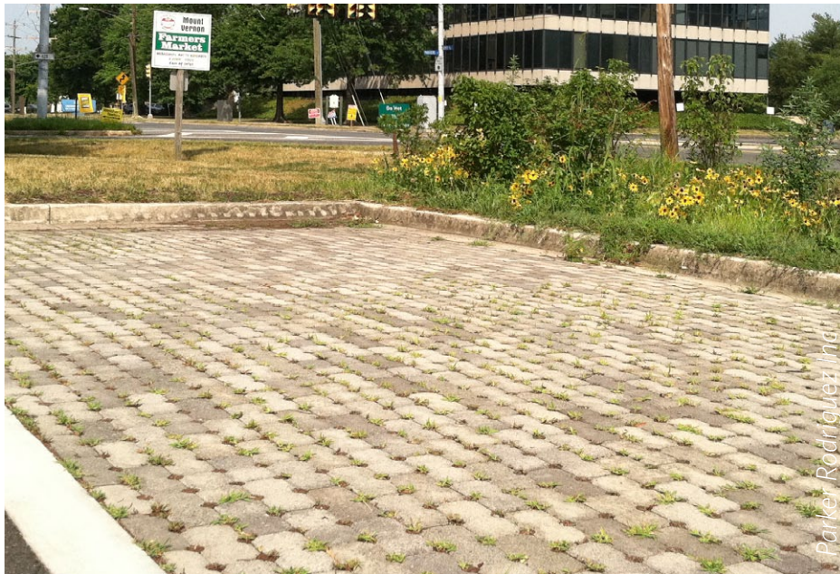
Figure 62: Sherwood Hall Library, Fairfax County, VA.
