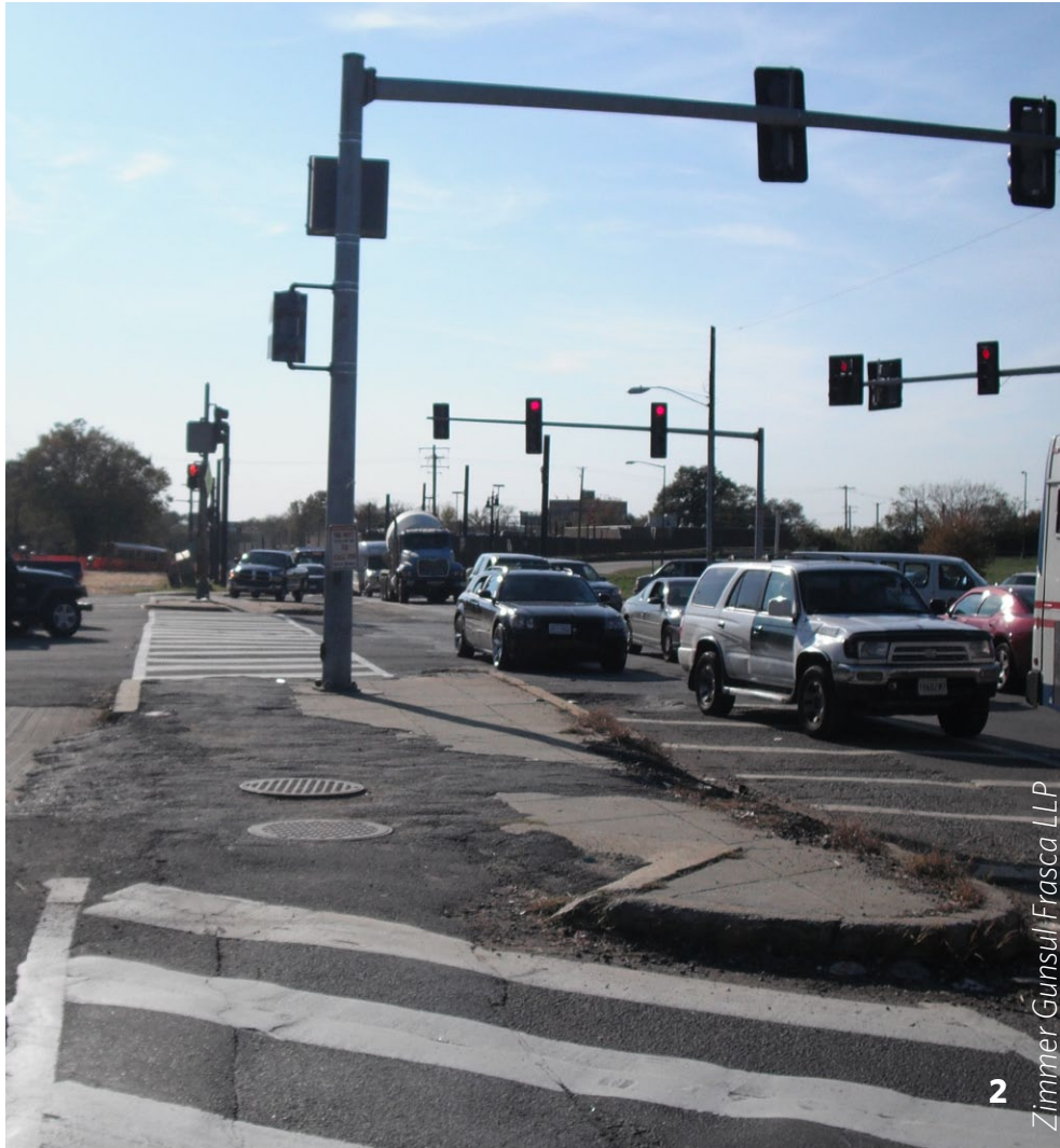
Figure 18: Though each of the free right turn lanes on Suitland Parkway has a small refuge, they are badly deteriorated and do not meet accessibility standards.
