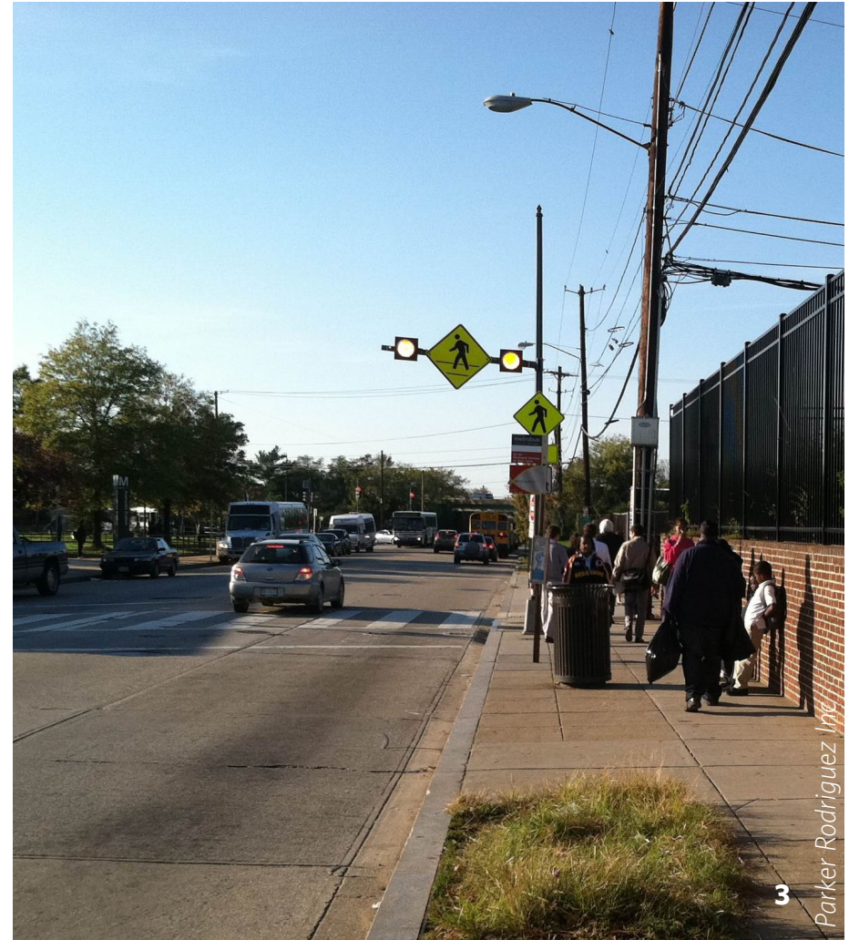
Figure 15: The crosswalk over Howard Road to the Anacostia Metro station from Shannon Place has a flashing yellow light to warn vehicles of pedestrians crossing. However, the sensor often does not function properly, and drivers often fail to yield to pedestrians.
