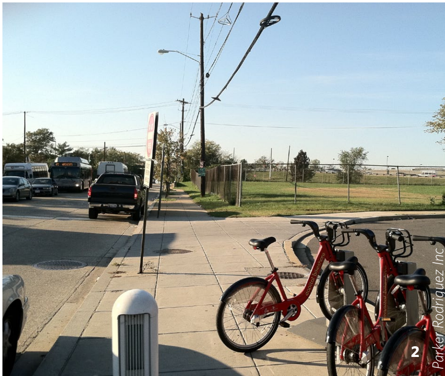
Figure 14: A rolled curb on Howard Road at Shannon Place allows emergency access, but many motorists drive over the sidewalk, endangering pedestrians.
