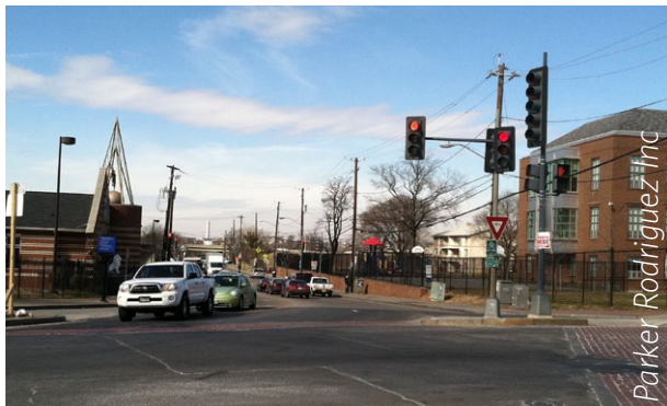
Figure 41: Current condition of Howard Road.
