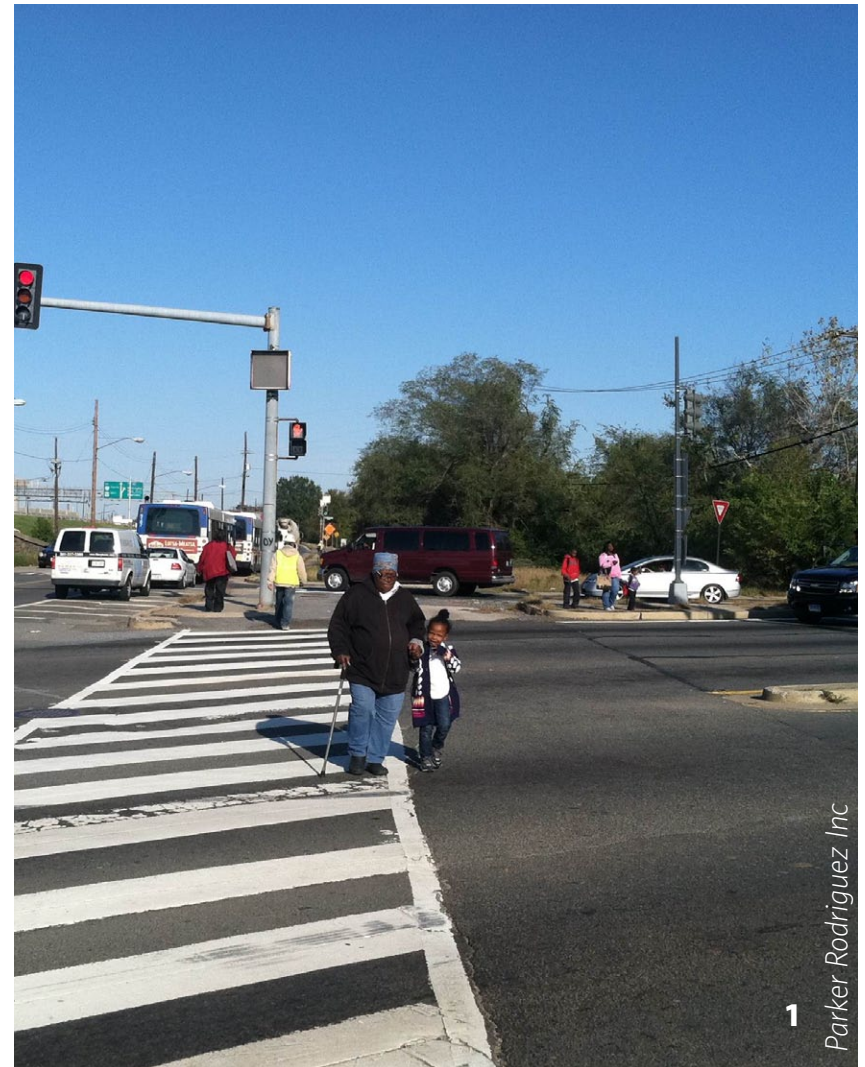
Figure 17: The crosswalk across Suitland Parkway is over 70 feet wide with no pedestrian refuge in the median and two free right turn lanes that allow drivers to turn right without slowing.
