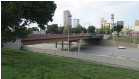
Figure 37: Existing View (Bridge over Interstate 630, from southeast).
