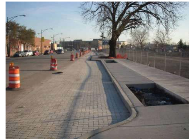
Figure 61: Cermak Road after construction of permeable parking/bike lane, stormwater storage, and sidewalk planters.
