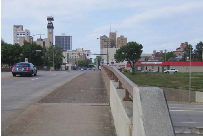
Figure 2: Main Street (at the I-630 overpass) as experienced on the design team's tour of the City.
