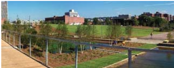
Figure 67: The Railroad Park site showing stormwater infrastructure.
