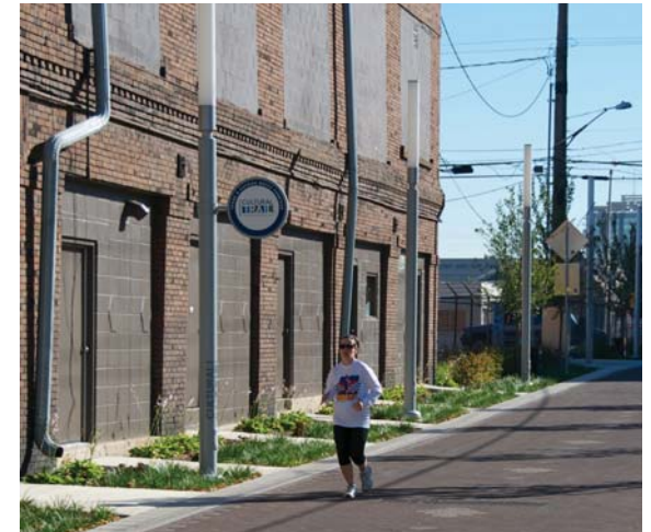
Figure 66: Downspouts flow into stormwater basins along the Trail.
