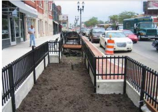
Figure 54: Michigan Avenue during construction.
