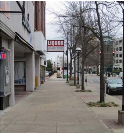
Figure 47: Existing view (Main Street, looking north from 4th).
