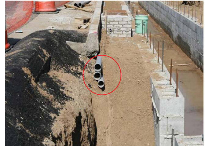
Figure 55: Construction photo showing utility conduits.
