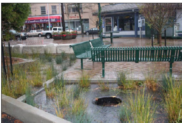
Figure C-13. Sheet flow of stormwater runoff enters a stormwater swale from a public plaza.
