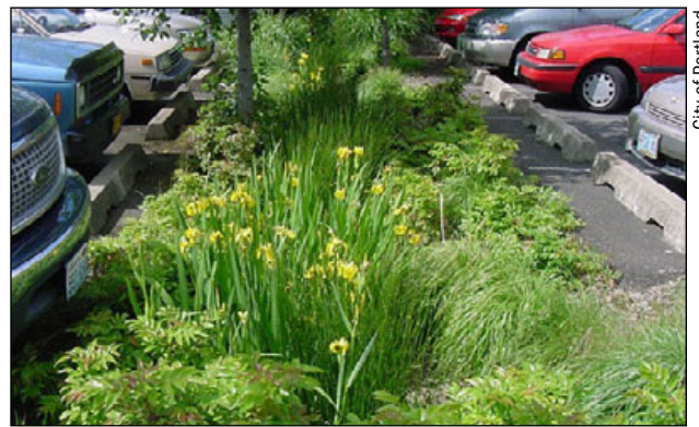
Figure 94. Parking lot swale with sheet flow between parking wheel stops.
