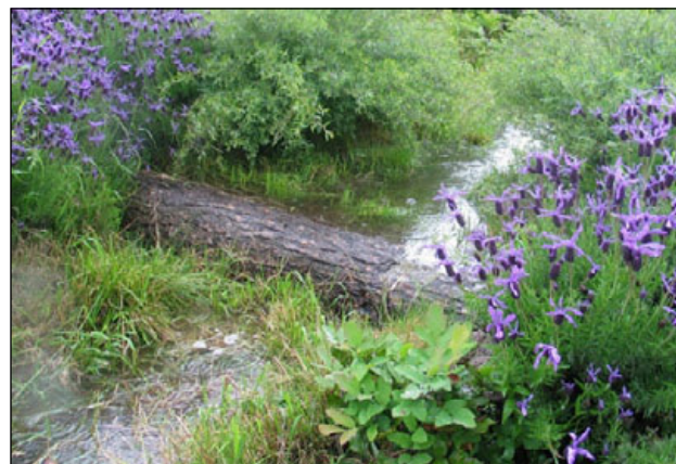
Figure C-29. Log check dam.
