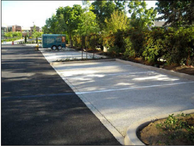
Figure 62. This parking lot uses pervious concrete in the parking stalls.
