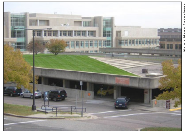
Figure 67. Green roof on a parking garage.
