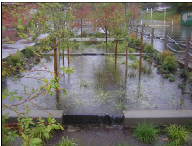
Figure C-26. Concrete check dam with an adjustable weir.
