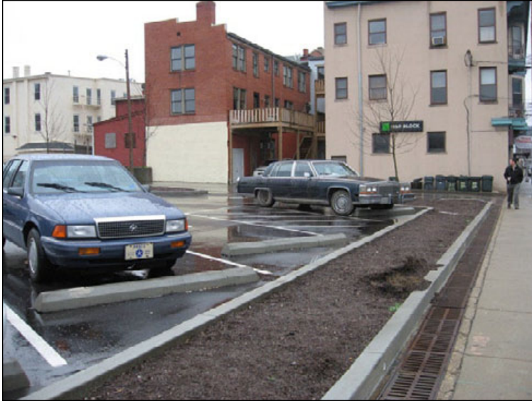
Figure 113. Angled parking creates an unused space between the wheel stop and the edge of the planter strip.
