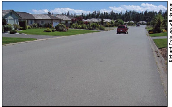
Figure 25. This street could be narrowed to create space for rain gardens and sidewalks.
