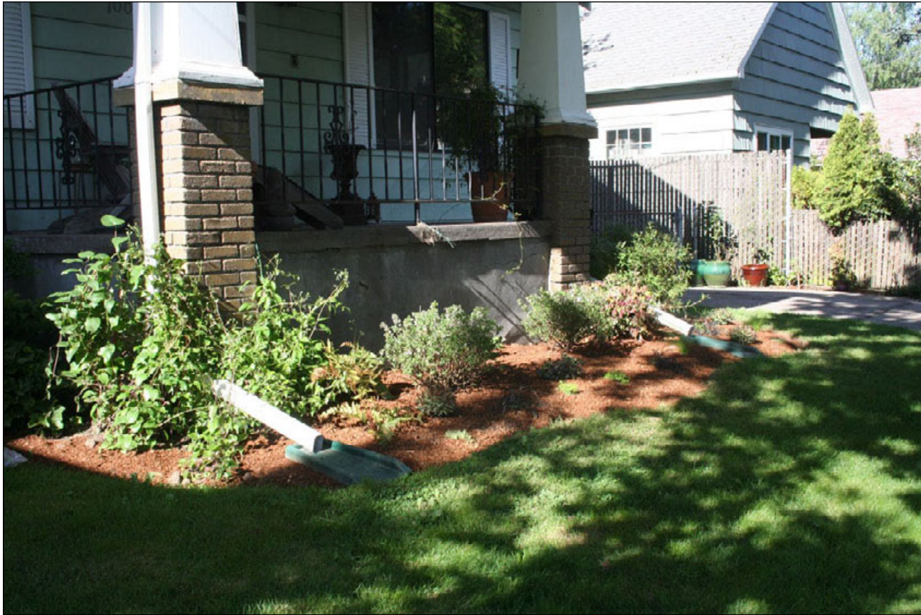
Figure 137. A disconnected residential downspout.
