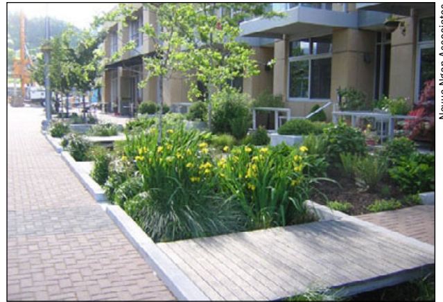
Figure C-5. Bridges over stormwater facilities allow access and maximize space to manage runoff.
