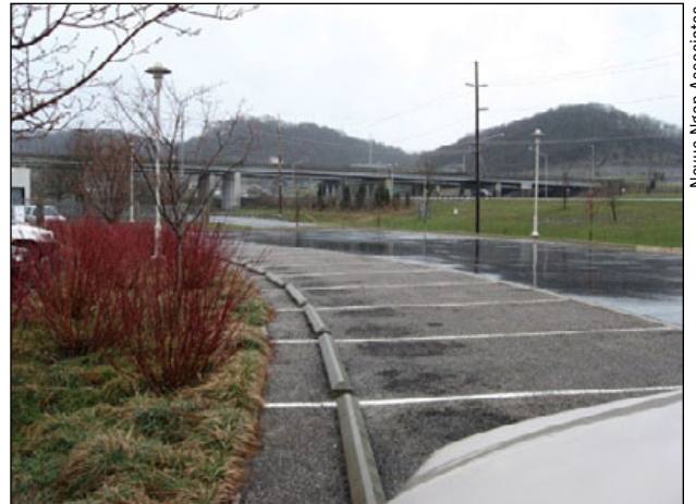
Figure 44. A pervious asphalt parking lot. The force applied by tires at turning, stopping, and starting locations can be hard on the paving surface.
