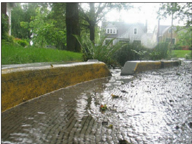
Figure C-12. A typical curb cut allows water to enter a curb extension.
