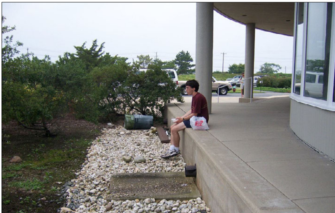
Figure D-2. Downspout disconnection into an infiltration garden at the University of Delaware's Lewes Campus.
