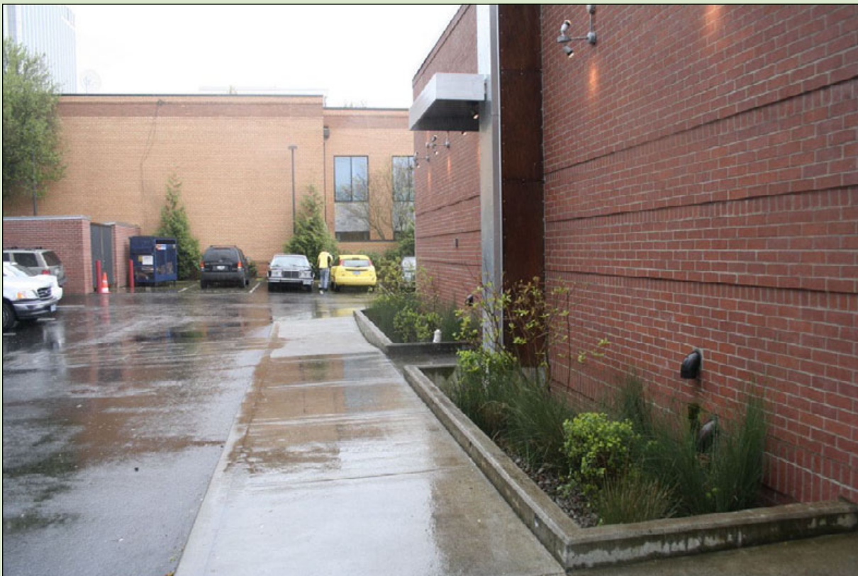
Figure D-4. A building flow-through planter accepts runoff from a fast-food restaurant in Portland, Oregon.
