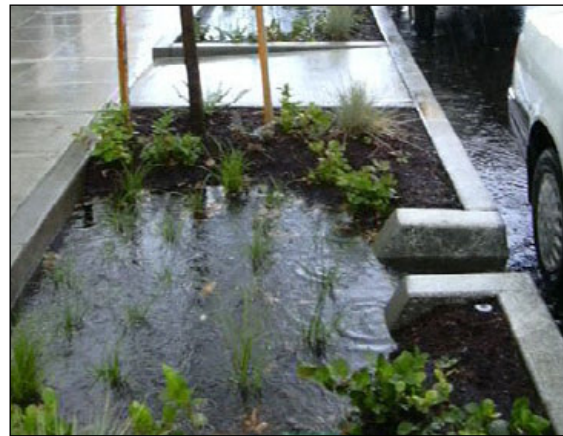
Figure 103. Stormwater planters accepting runoff from a commercial street.
