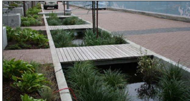
Figure 81. Stormwater swale in a mixed-use community. Boardwalks link pedestrians to the sidewalk zone of the street.
