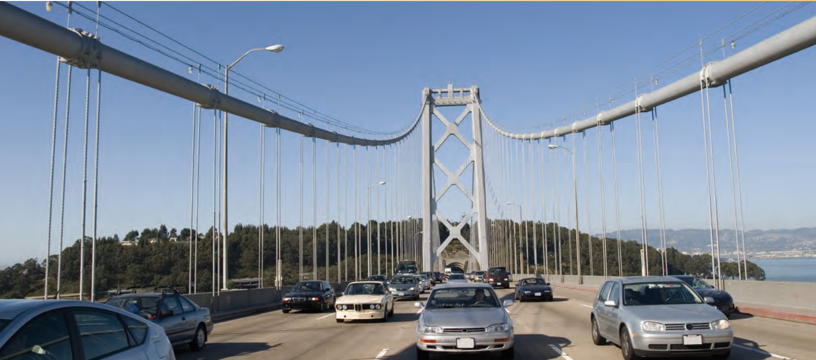
Bay Bridge in San Francisco, California
