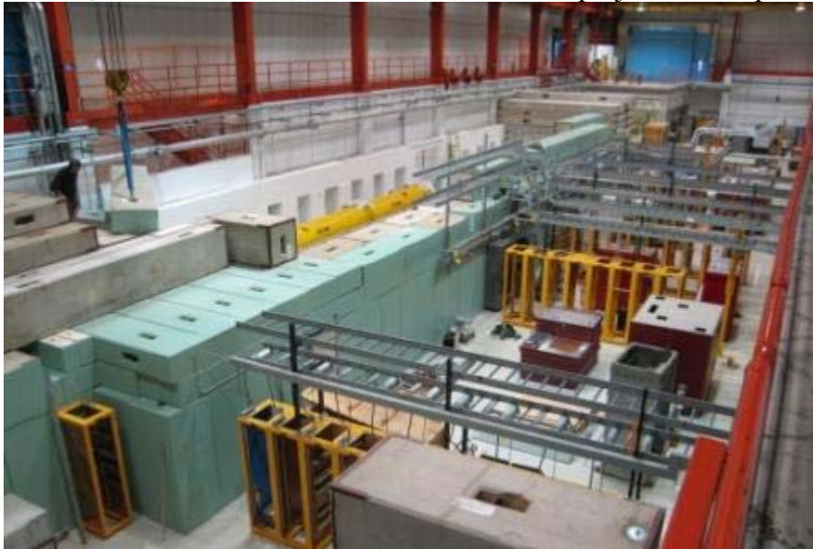
Figure 5.1: Photograph of interior of NML building, looking towards future high energy end. Visible is a single cryomodule (yellow).
