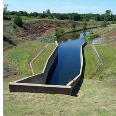
River outlet works, Fort Cobb Dam.
