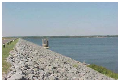
Fort Cobb Dam and Reservoir.
