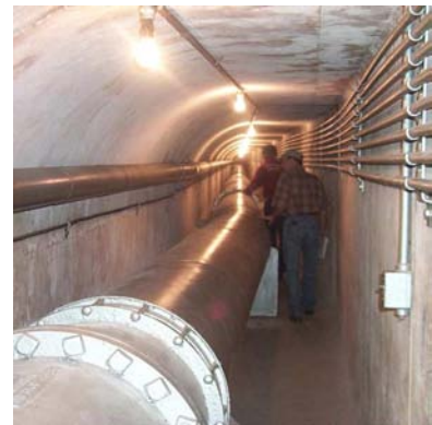
Anadarko Aqueduct inside Fort Cobb Dam.
