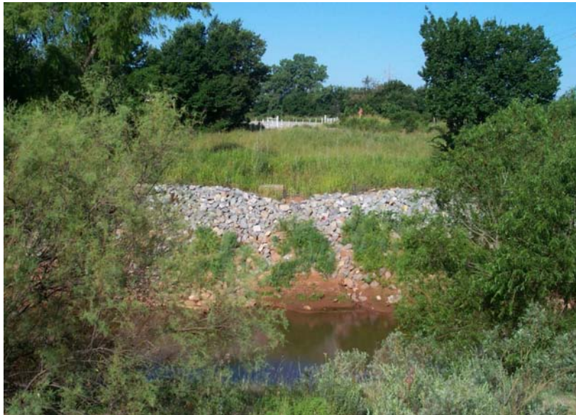
Maintained right-of-way of the Anadarko Aqueduct. A rip-rap protected stream crossing is in the foreground.
