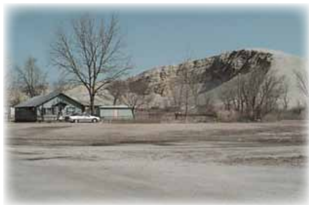
Tar Creek House Located Adjacent to a Chat Pile
