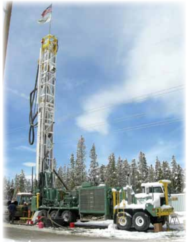
40-Foot Drill Rig Used to Reach Tunnel in Leadville, Colorado
