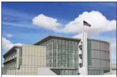
New Nebraska National Guard Joint Force Headquarters.
