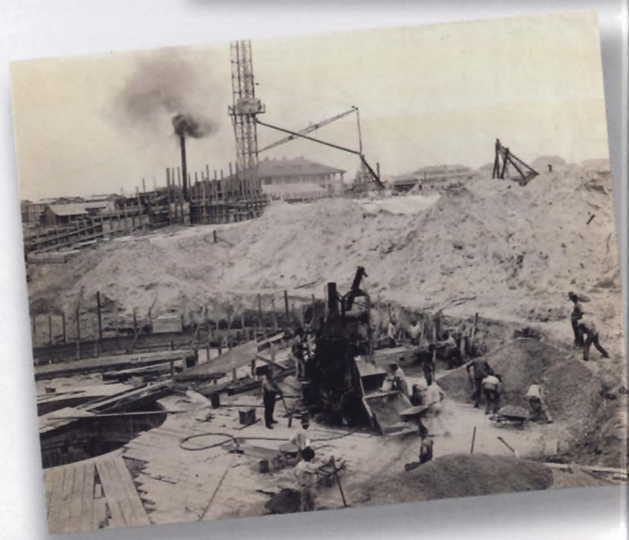
Galveston seawall construction, 1918. RG 77
