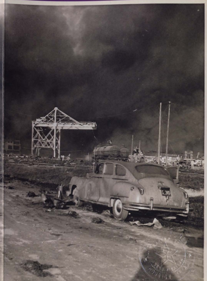
Damage from fire and explosion, Texas City Disaster, April 16, 1947. RG 21
