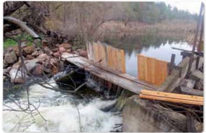
Exhibit 15: Grenada Irrigation District Dam, 2009. Photo courtesy of Bob Pagliuco.
