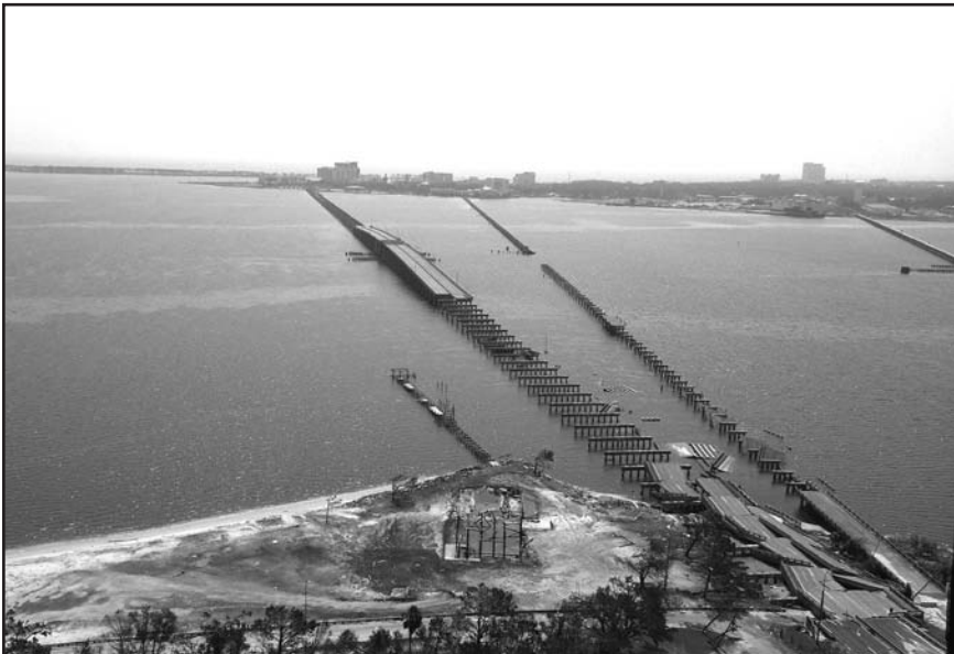
Figure 15. Damage to the Ocean Springs Bridge.
