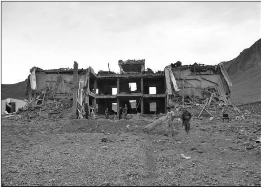
Figure 6. The Wreckage of the Musahi District Government Center.
