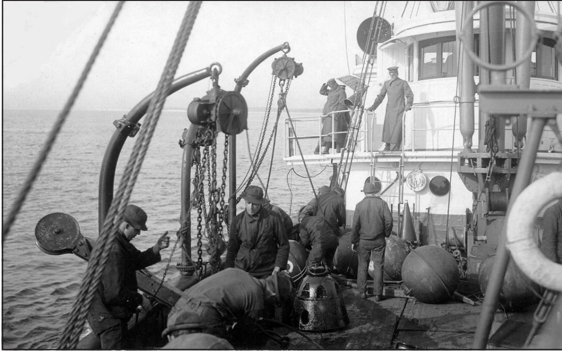
U.S.A.M.P. Royal T. Frank conducting mine planting operations near Fort Pickens, FL.
