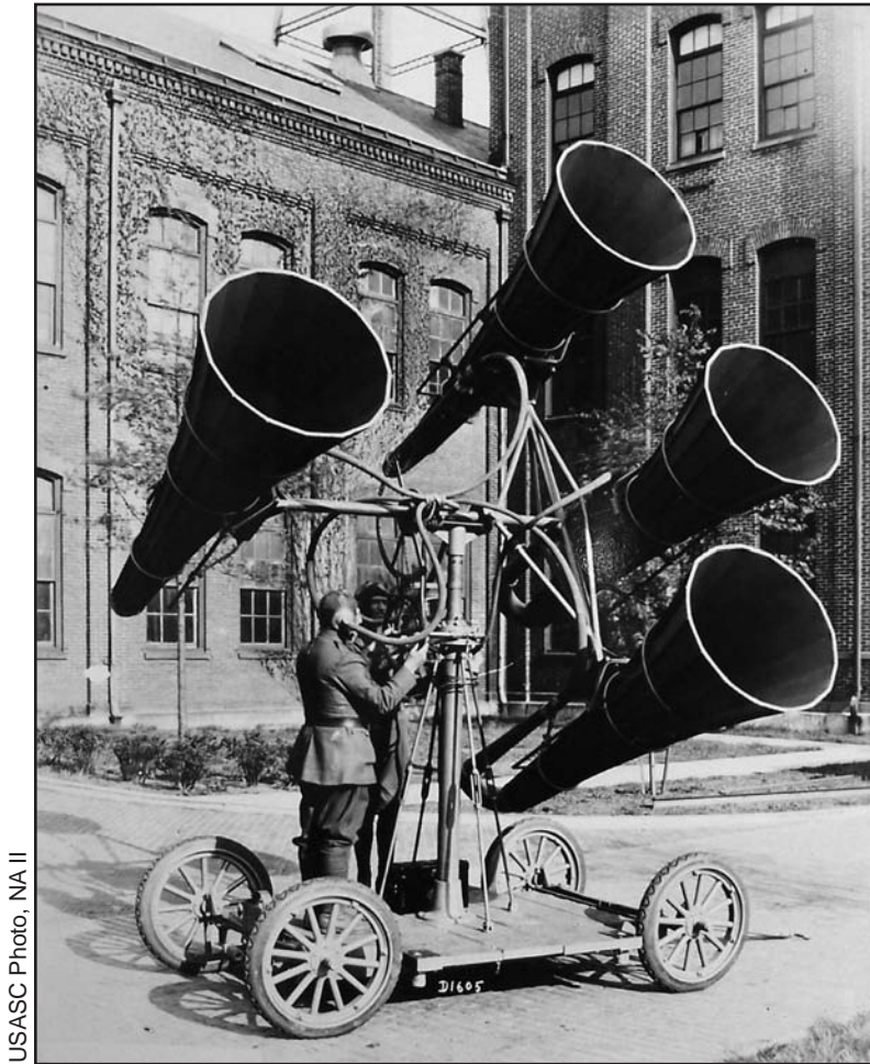
Soldiers conduct training on a sound detection system, circa 1925.
