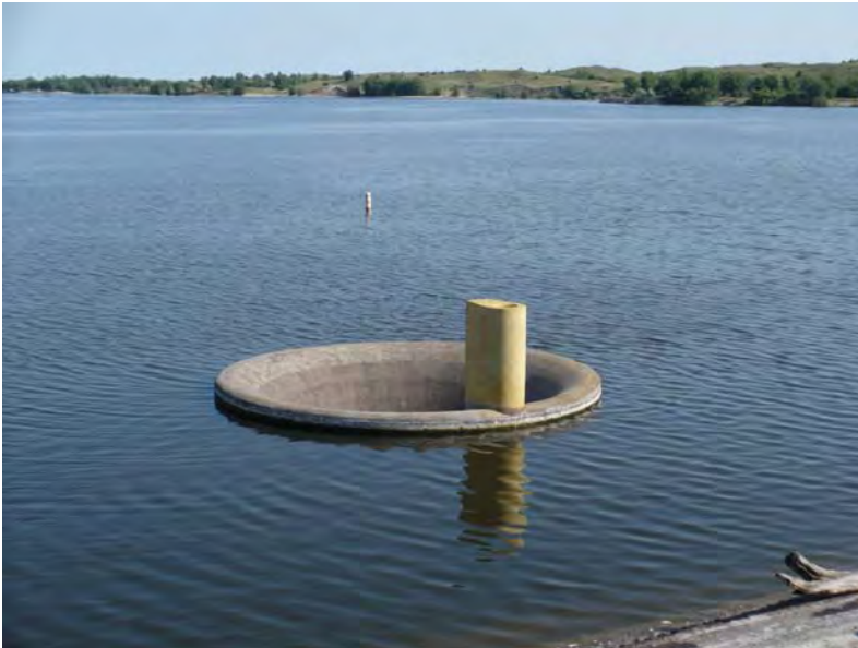
Figure 19 – Morning Glory Structure – Uncontrolled Spillway.
