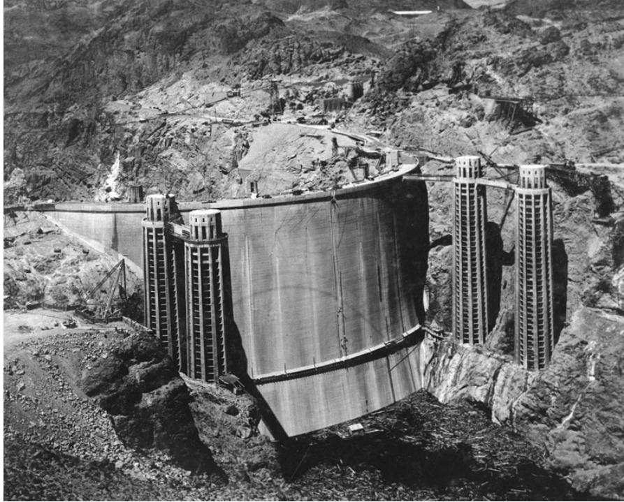
Figure 5 - Upstream face of Hoover Dam and four intake towers.
