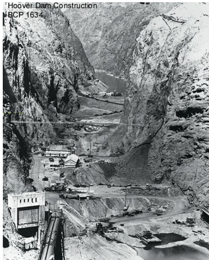
Figure 6 - Hoover Dam cofferdams.
