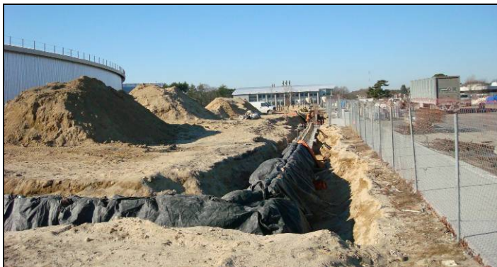
Figure 3: Foundation work for the Lab-Office Buildings.
