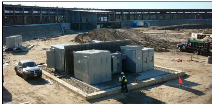
Figure 5: Punchlist items are being addressed.
