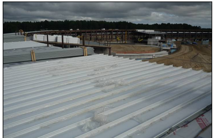
Figure 8. Pentant 1 standing seam metal roof being installed.
