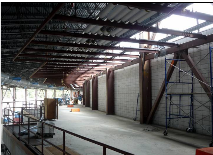
Figure 7. RF area masonry wall seen the from electrical mezzanine. Installation of the railing and stairs is complete, and masonry wall block finishing is in progress.
