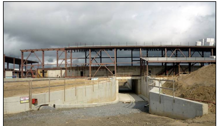
Figure 5. Vehicle tunnel being readied for use during construction.
