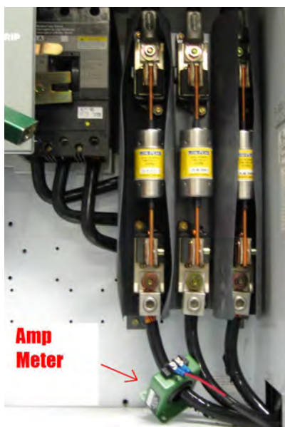
Amp meter used at a Trenton, Michigan, plant to gather data on electrical usage.
