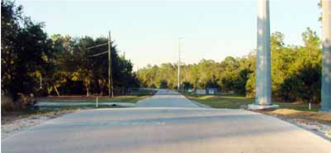
Figure 9. Photograph of accident highway-rail grade crossing.
