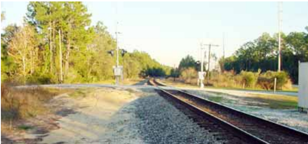
Figure 10. Photograph of accident highway-rail grade crossing.
