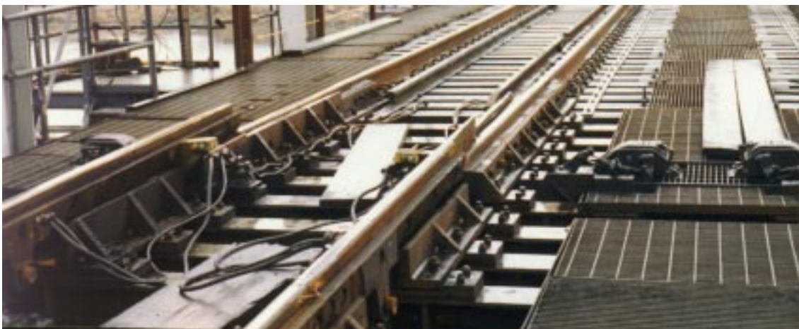
Figure 5 — Looking west along track 1 with miter rails in the lifted position
