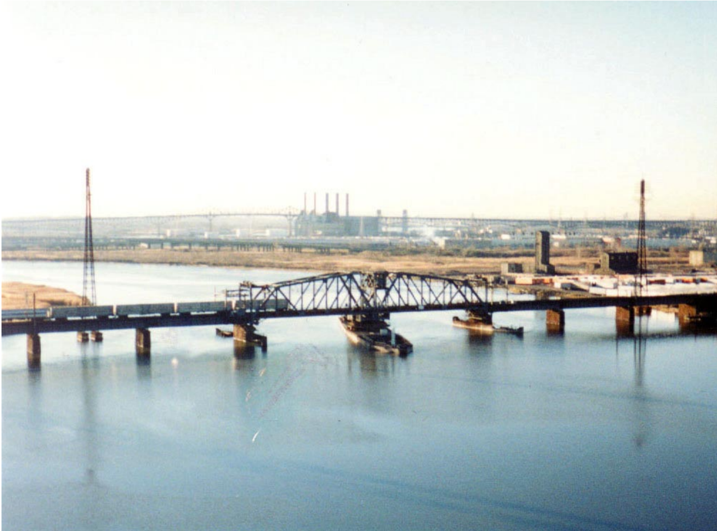
Figure 1- Looking south over Amtrak's Portal Bridge spanning the Hackensack River near Secaucus, New Jersey
