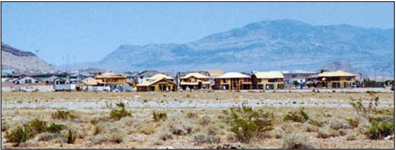
Housing construction in the Summerlin Master Planned Community, built by the Howard Hughes Corp., in western Las Vegas on the border of the Red Rock Canyon National Conservation Area.
