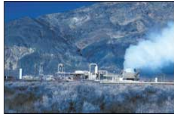
Caithness Power Inc. geothermal power plant in Dixie Valley, Nevada.
