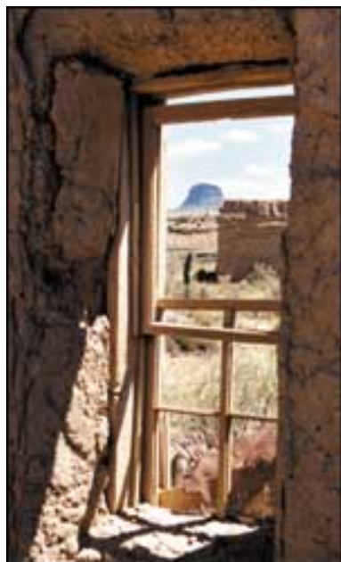
An old adobe ruin gives a picturesque view of Cabezon Peak Wilderness Study Area in the town of Guadalupe, New Mexico. Photo by M'Lee Beazley
