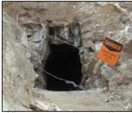
Mine entrance on the edge of Las Vegas. BLM-Nevada is working to reduce many such hazards to users of public lands.
