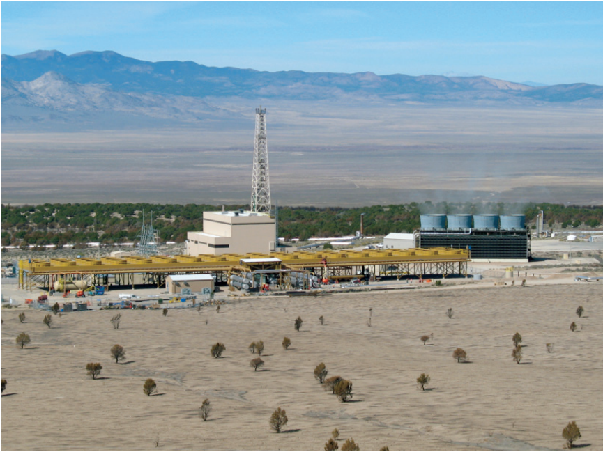
Figure 5. The Blundell geothermal power plant at Roosevelt Hot Springs, Utah (Photo: R. Blakett)
