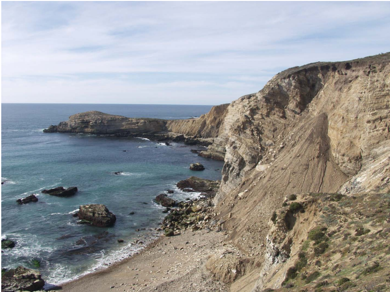
Figure 3. Landslide at Weaner Cove
