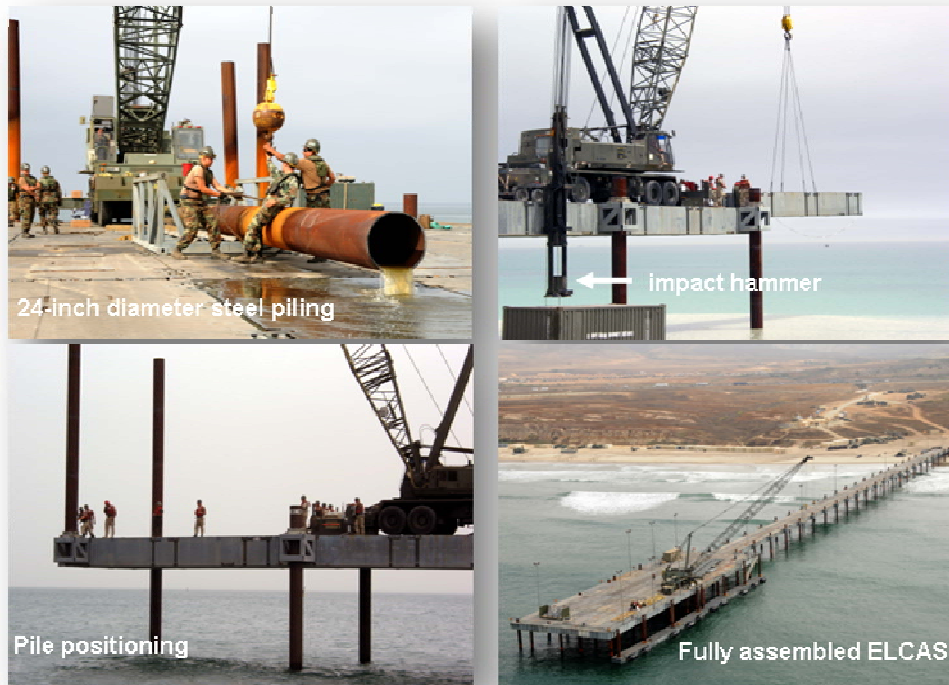
Figure 1-3. ELCAS construction stages.
