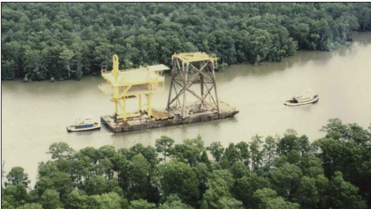
Figure 1-15. Four-Pile Jacket, Topsides, and Components (TENNECO ST59 “A”) Sea-Fastened to a Load Barge on Route to Morgan City, Louisiana, for Recycling and Scrapping (MMS Staff Photo).
