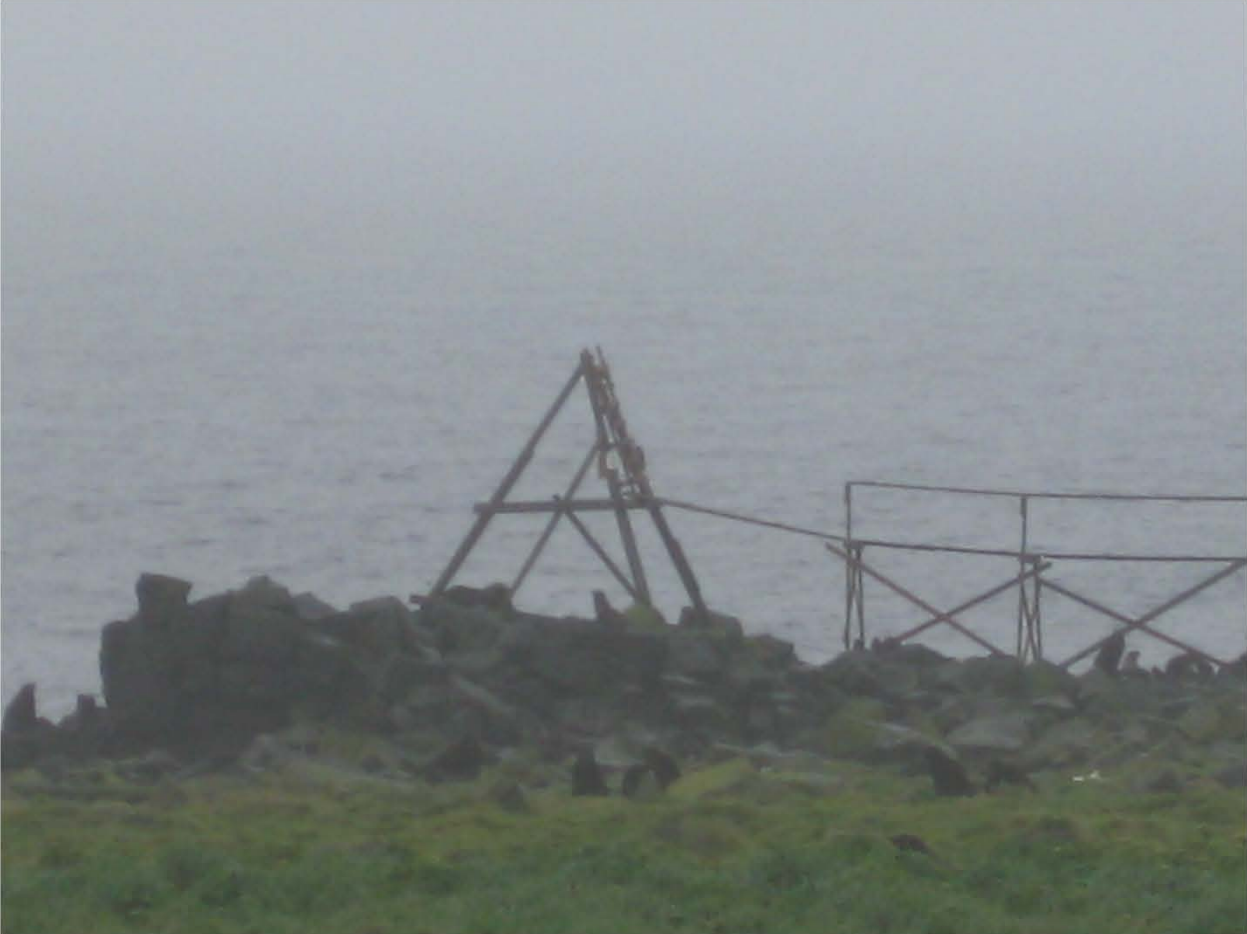
Example of an existing observation structure.
