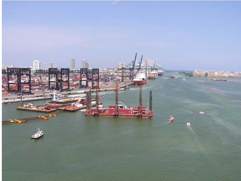
Figure 2. Drill Barge Apache set up in Miami Harbor.
