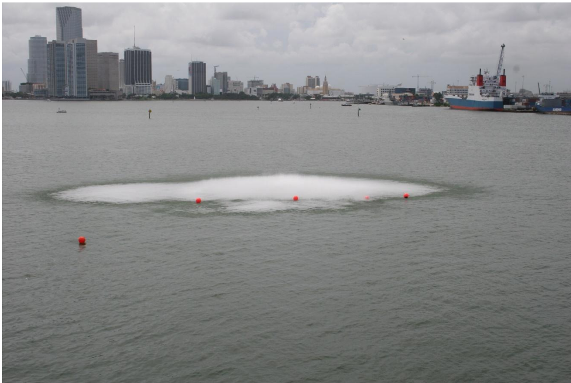
Figure 10 – (Figure 9 of the ACOE’s IHA application) Confined blast of 3,000 lbs total charge weight of explosives.
