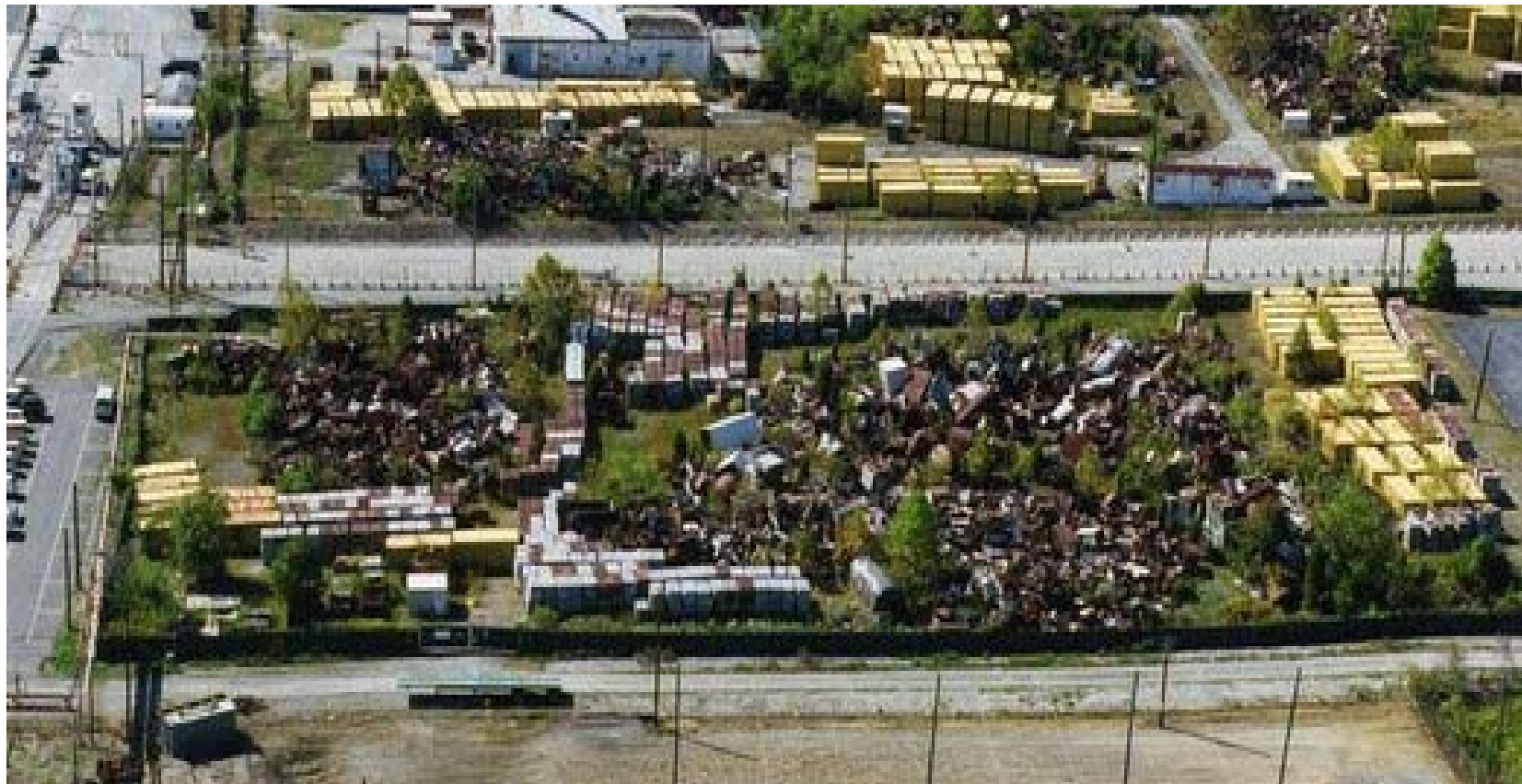
Old Scrap Yard Prior to ARRA Work Progression
